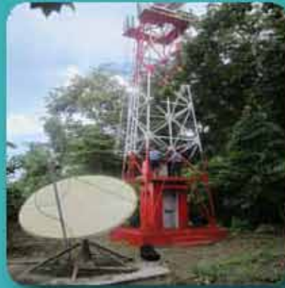
Director General of Lighthouse and Lightship- Automation equipment installation at Wilson Island, Andaman and Nicobar Islands
